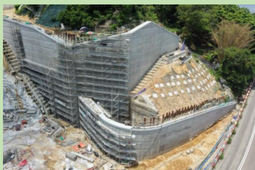
擋土牆混凝土結構工程 Concreting Works for Retaining Wall
