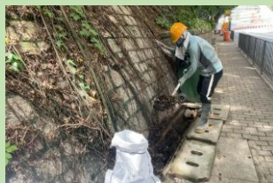
清理排水設施 Clearing the Existing Drainage Facilities
