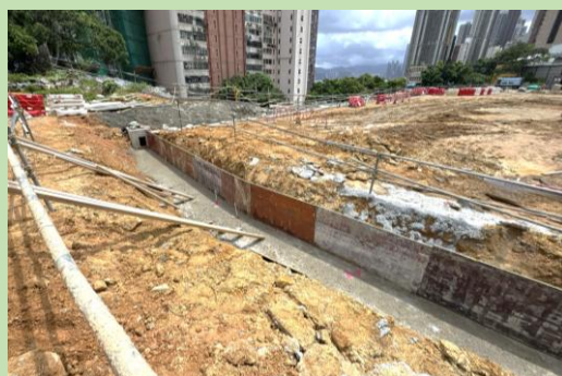
渠務工程 Drainage Construction Works
