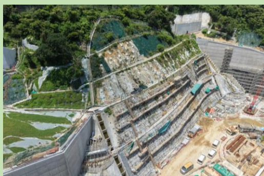
斜坡鞏固工程 Slope Stabilizing Works
